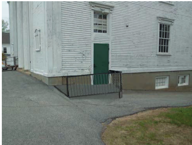
Conceptual photo rendering of the lowered side door to allow for wheelchair access to a lift behind.
